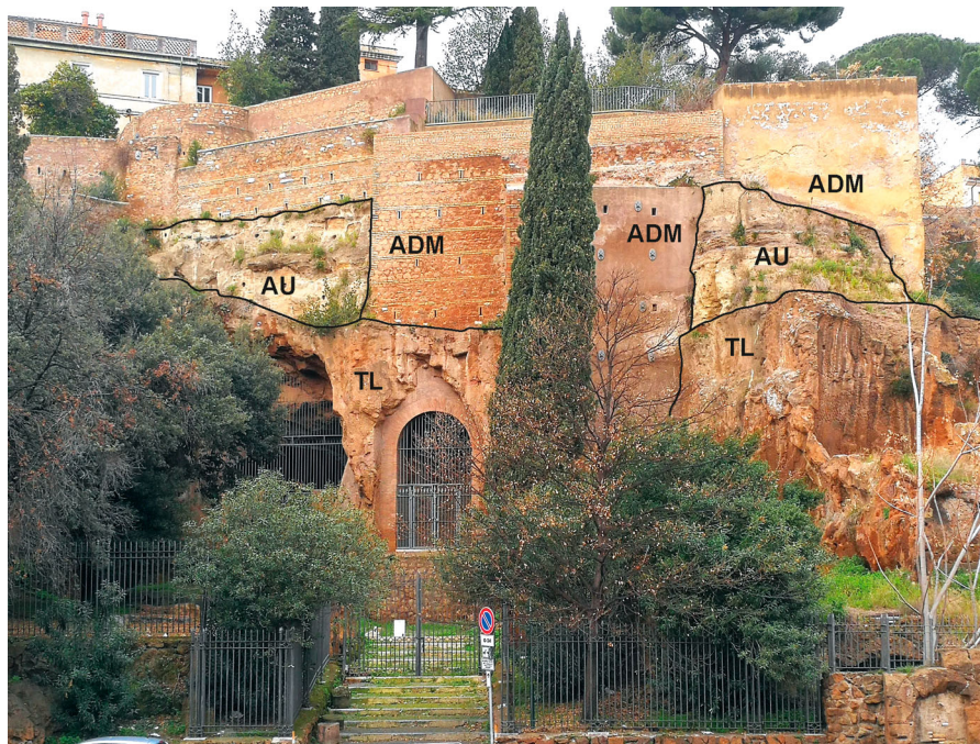
Figure 4. The southern flank of the Capitulum, photo taken from piazza della Consolazione. From the street level, the middle of the image displays the entrance to one of the huge underground quarries ( latomie ) operated during the ancient Roman age to provide lithic pyroclastic blocks useful for construction. The steep slopes resulted from both topple landslide processes and from anthropogenic erosion. Legend: ADM – Anthropogenic deposits and materials (retaining walls and foundations of the buildings), covering natural deposits also in the lower portion of the image; AU – Aurelia Unit fluvial-lacustrine deposits (Middle Pleistocene); TL – Tufo Lionato pyroclastic-flow deposits (Middle Pleistocene).
