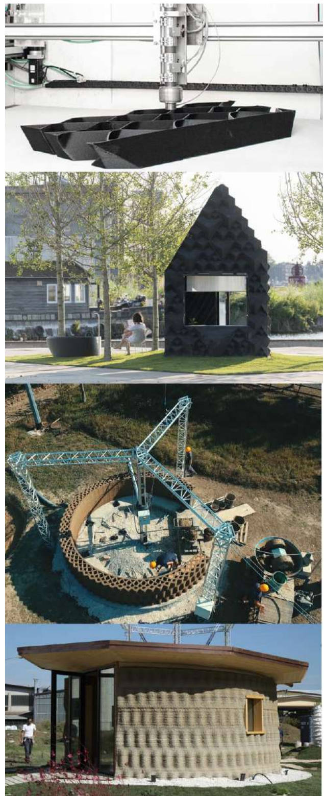
Fig. 1: Experimental projects illustrating the two principal strategies for using 3D printing technologies. Urban Cabin by AECTUAL (2015) realised in formwork 3D printing (© Sophia van den Hoek, AECTUAL). Below: Gaia by Wasp (2018) produced by direct 3D printing. (© WASP)
