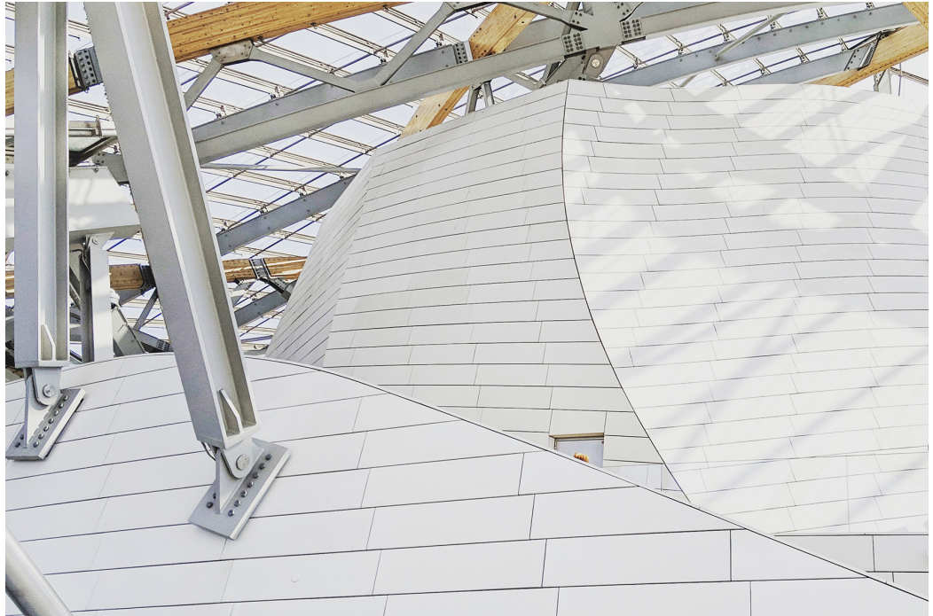
Fig. 5. The fiber-reinforced concrete panels of Louis Vuitton Foundation designed by Frank O. Gehry in 2014.
