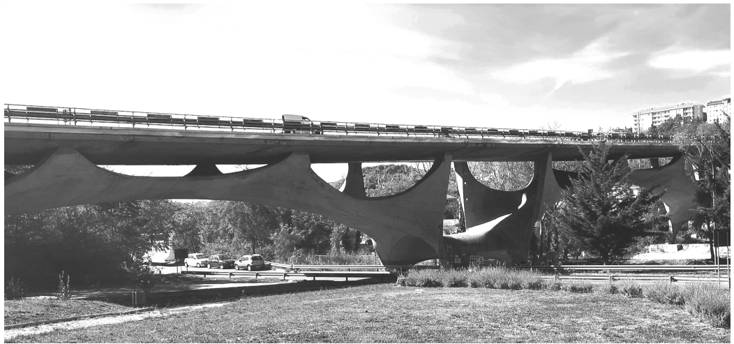
Fig. 3. Bridge over the Basento river designed by Sergio Musmeci in 1967.
