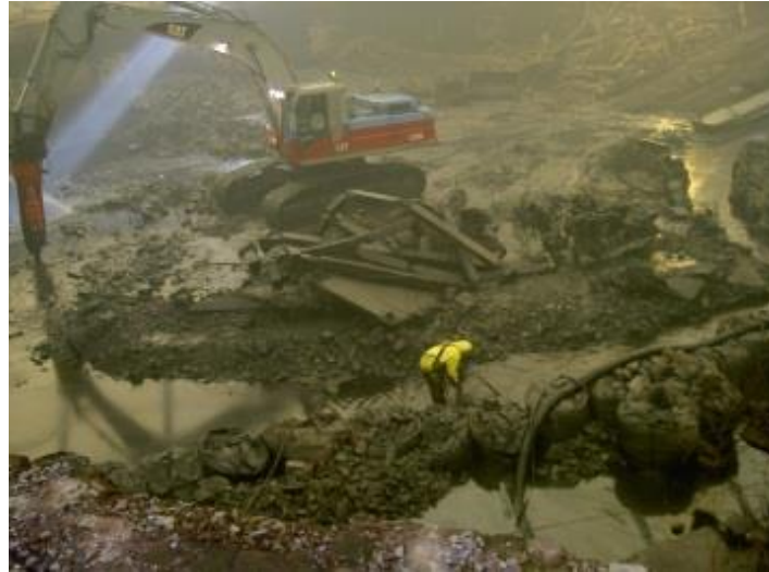
Figure 16. Gustafson, Porter and Bowman, Cuulturpark Westgasfabrieck. A new public park designed on the heavily contaminated gas factory site. Contaminated soil could not be removed and transported elsewhere. The placement of the contaminated soil on-site was the best environmentally economical oriented decision. 2006 Amsterdam.
