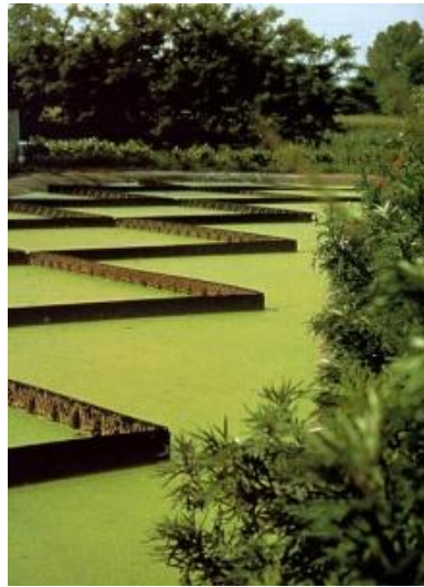
Figure 2. Viet Ngo applied his method, Lemna System, of water's treatment and purification in the Molgora River that looks like a land-art installation, Adda affluent, in north-west Italy, 1990.
