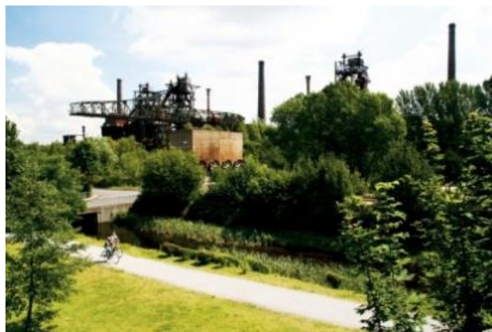
Figure 11. Latz und Partner, Landschaft Park. Peter Latz’s strategy focused on remediation through either isolating the contaminated dirt in bunkers on site or leaving it in place, allowing it to improve in quality through phytoremediation, where plants are used to contain, degrade and eliminate contaminants in the soil through their roots. Duisburg Nord 1991–1998.
