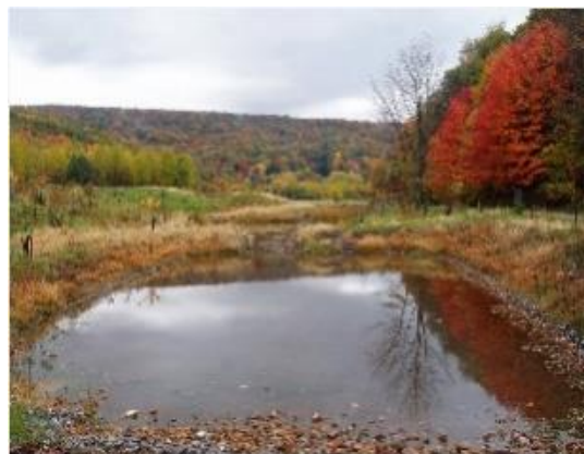
Figure 4. AMD&ART. Acid Mine Drainage through a passive treatment system, relying on natural processes to raise the pH and remove the metals. This type of system has several benefits, including low overhead and maintenance costs. Passive treatment systems also provide more design opportunities, and can create new opportunities for historical, natural and scientific understanding. Vintondale, Pennsylvania, 1995–2004.
