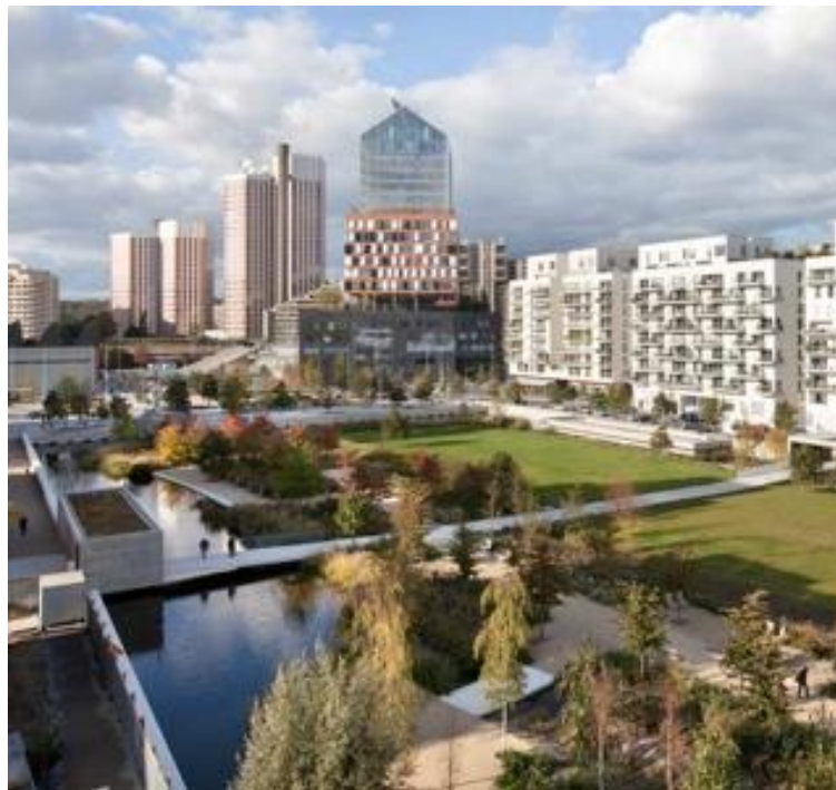
Figure 24. Trapéze park in Boulogne Billancourt is at the heart of the district’s rainwater management system. The permeability of its soils and the storage of water in hollow gardens filters all rainwater which is then partially recovered in a basin to be reused for irrigation.
