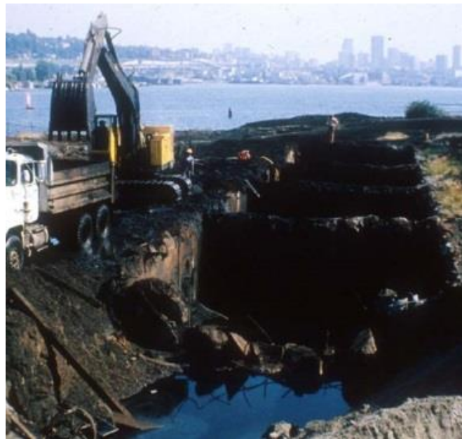
Figure 9. Richard Haag, Gas Work Park. Soil treatment on the former Gas Plant. Work on site was experimental, for the first time involving bioremediation and biodegradation of dissolved organisms present in the soil. Seattle, 1970–1975.
