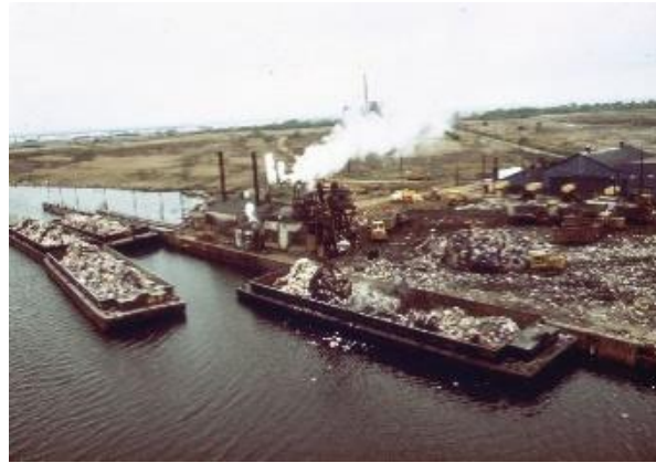
Figure 5. Fresh Kills opened in 1948 as a temporary landfill and it remained so until its closure in 2001. At the peak of its operation, in 1986, it received 29,000 tons of residential waste per day. In the picture is the landfill in 1974.
