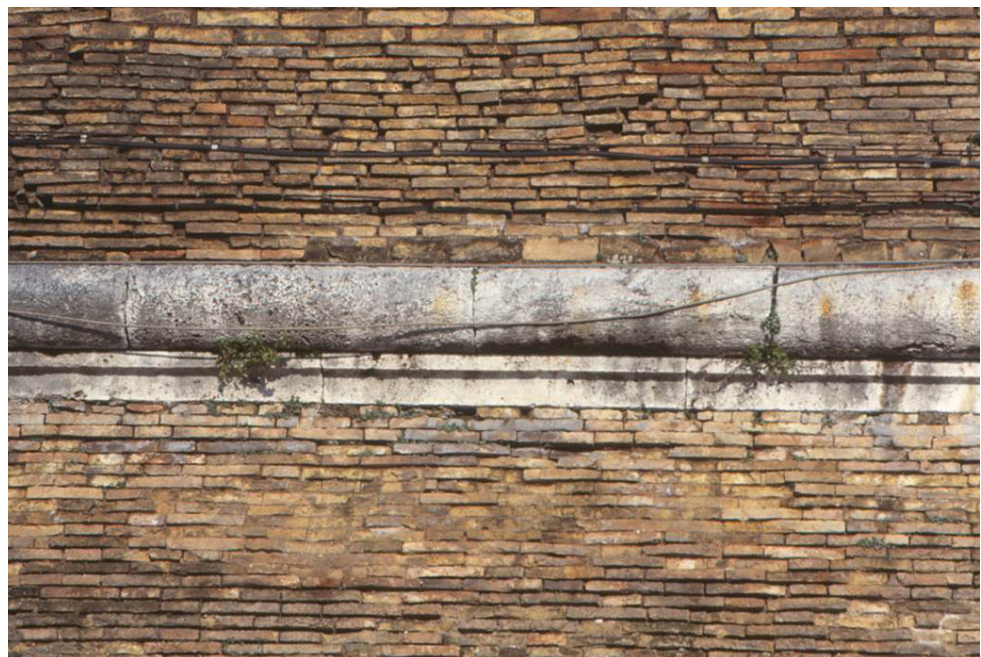
Fig. 19. Detail of the bastion's masonry, made of brick with the toro . Photo by C.B. 1985.
