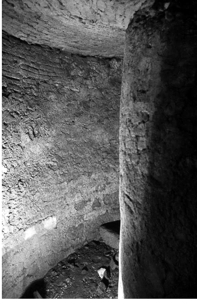
Fig. 25. Detail of the helicoidal ramp. Photo by C.B. 1985.
