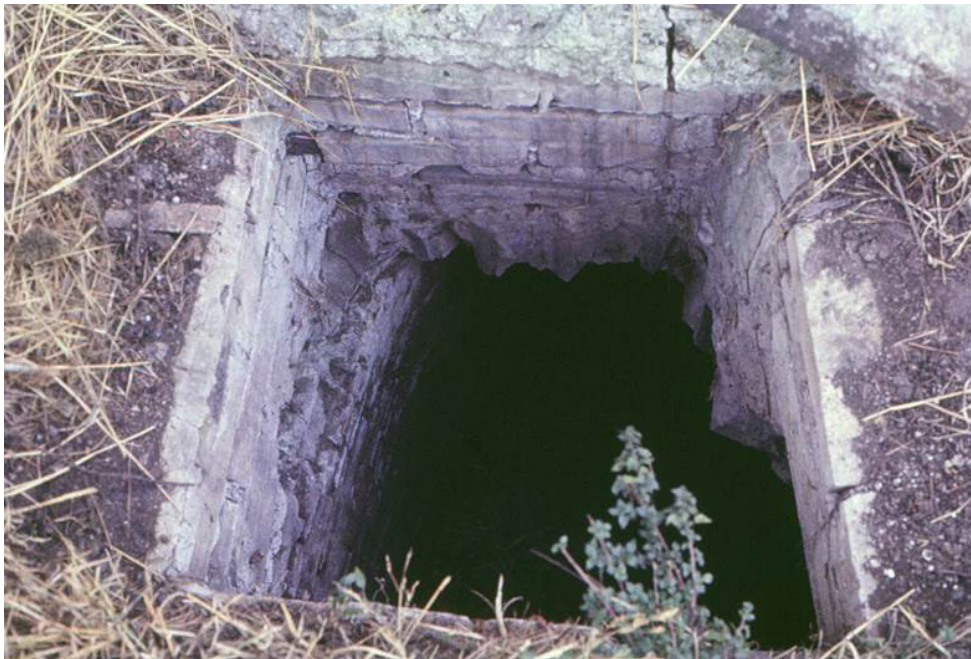
Fig. 24. Photo of the “trap door” that allows the entrance from the top of the vault, discovered after the melting of the snow. Photo by C.B. 1985.
