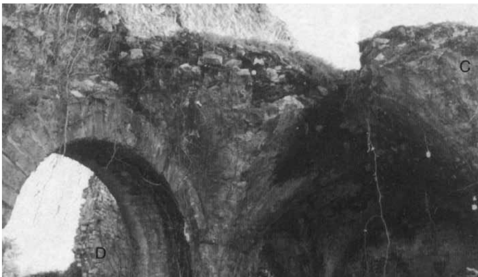
Fig. 26. Ninfa, San Pietro, ruins with the constructive detail of an extradosed vault.
