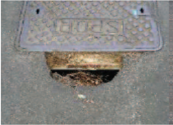
Fig. 10 – An example of poorly maintained sidewalks, in the home-to-school path near Piazza Mincio.
