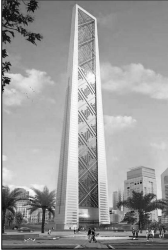
5-4 The Lighthouse Tower, Dubai
