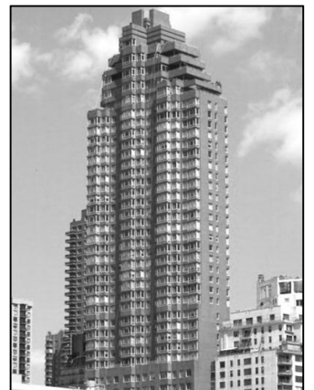
4-9 Belair residence in NY
