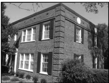
1-5. Colonial Village Apartment Gustave Rings first project in Arlington
