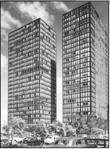
1-4. Lakeshore drive apartments by mies van der rohe; 1951
