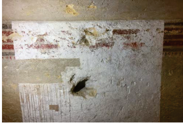
FIGURE 1. Picture of the unrestored part of Tomba Bartoccini , where the white patina is visible.
