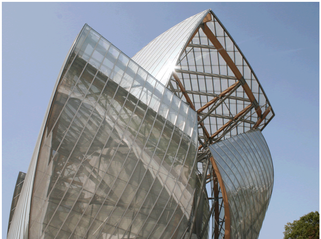
Fig. 8. Frank O. Gehry, Louis Vuitton Foundation, Paris 2014. Detail of the external envelope formed by single-curved surfaces divided into panels by adopting paneling procedures [Lanzara 2020 pp. 97, 98]. (Photo by the author).
