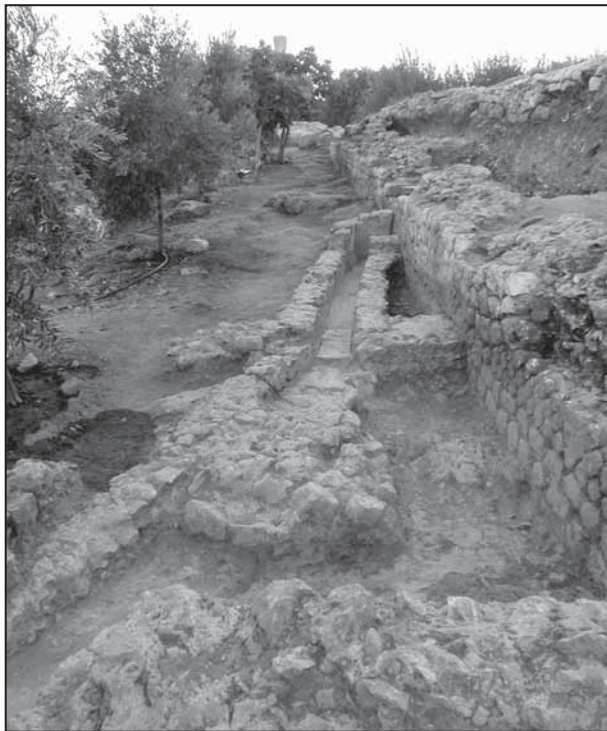
Fig. 8: Temple area: View of the east-west wall supporting the terrace north to the temple and of the channel system.
