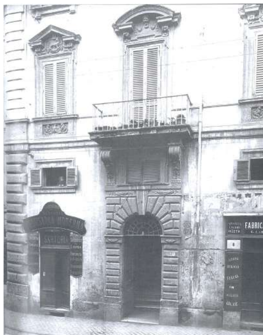
Fig. 2. Photograph of the building at n. 7 of Via Alessandrina before it was demolished [Delli 2007, vol. 1].
