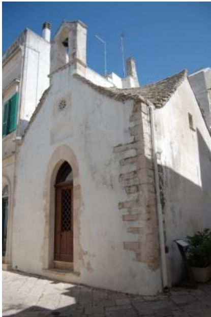
Figure 1. The Church of San Nicola in Montedoro
