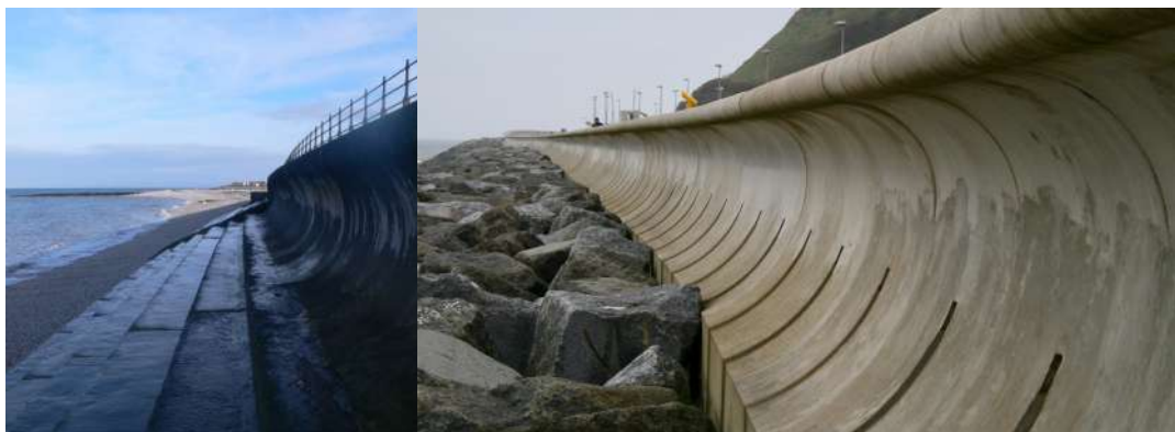
Figure 1. Wave return wall located in Penrhyn Bay, Great Britain reported in the left panel. Recurved seawall with rock armour at Scarborough reported in the right panel.
