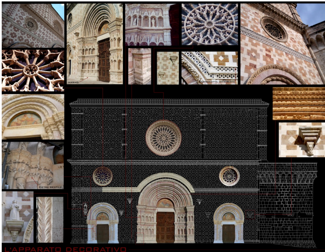
Fig. 9 Façade survey: the decorative system.
