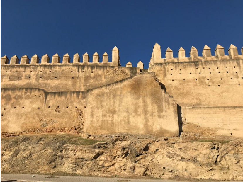
Fig. 4: The ancient walls of Fès, Place Boujloud.
