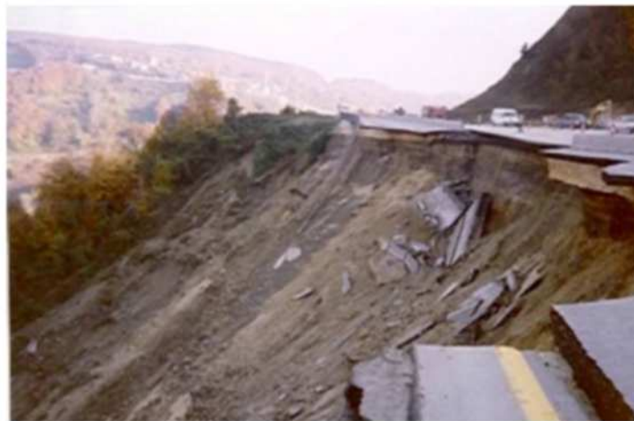
Figura 30 Frana sulla E5 Highway in Duzce Earthquake Report on 1999 kocaeli and düzce (turkey) earthquakes - Mustafa Erdi
