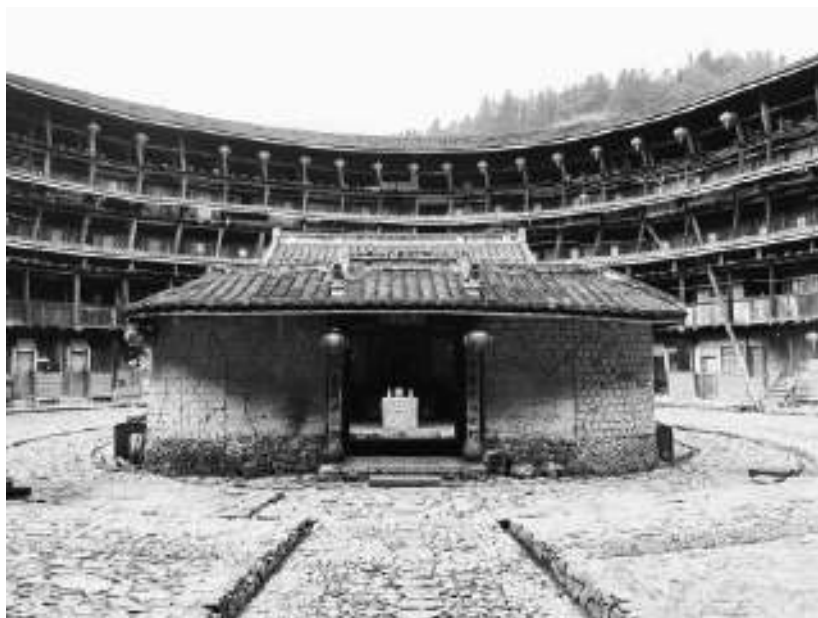
Fujian Hakka Tulou, Nanjing county: exterior and interior view of a circular-plan construction.
