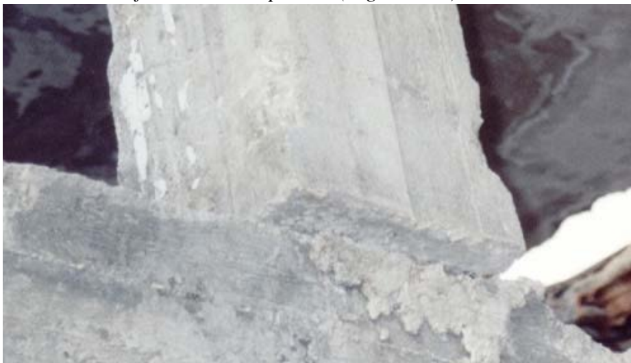
Figure 2.14: Fixed-end rotation at the base of column
