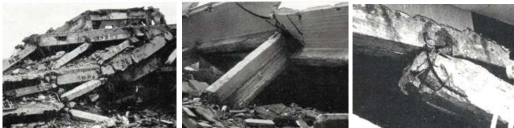
Figure 2.9: Irpinia earthquake (1980), the global collapse of an hospital building due to formation of a soft story and poor local details.
