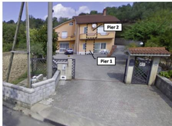
Figure 4.8: Structural components over the building façade
