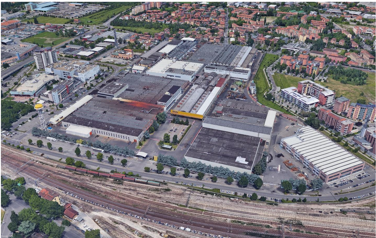
Figure 3. Industrial plant operating in north Italy.
