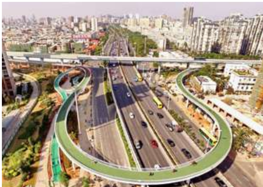
Dissing + Weitling, Xiamen Bicycle Skyway, 2016-2017 (foto di Dissing + Weitling)
