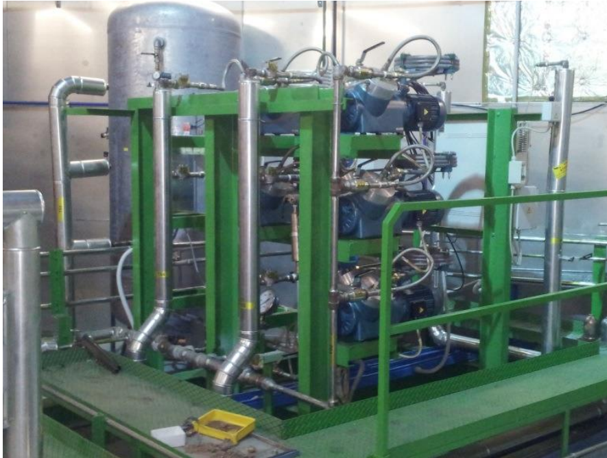
Fig. 2-3 – View of the compressor unit for the argon circulation
