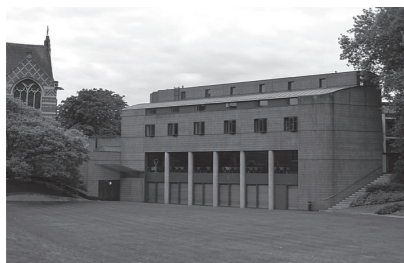
ARCO Building, Keble College, Oxford, UK
