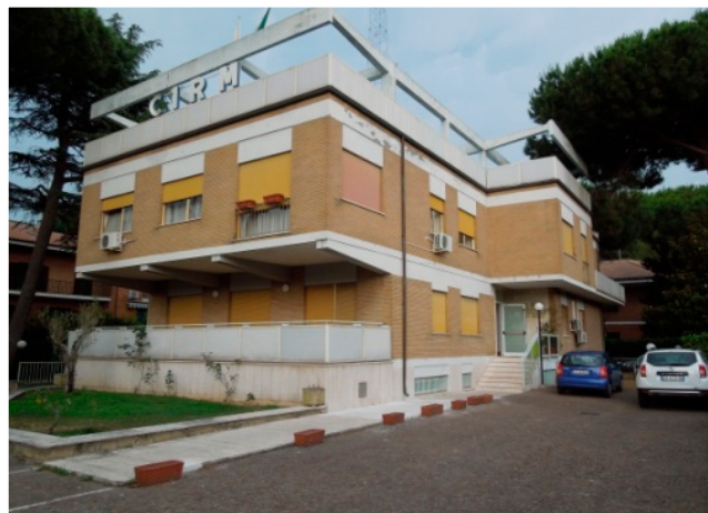
Figure 3. The International Radio Medical Centre (CIRM) administrative headquarter building.
