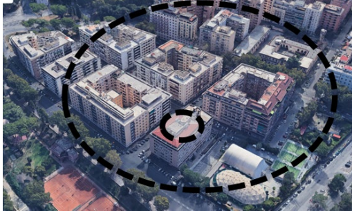
Figure 4. The measurement on a GS in high-density area of buildings can identify its membership to a GMS: the two circles D_p=32 m and D_{mes}=256 m show the equivalent areas of the sample case of ground electrode related to the resistance calculated and measured respectively
