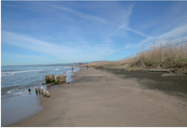
Fig. 8 - View of the backshore subjected to severe erosion
