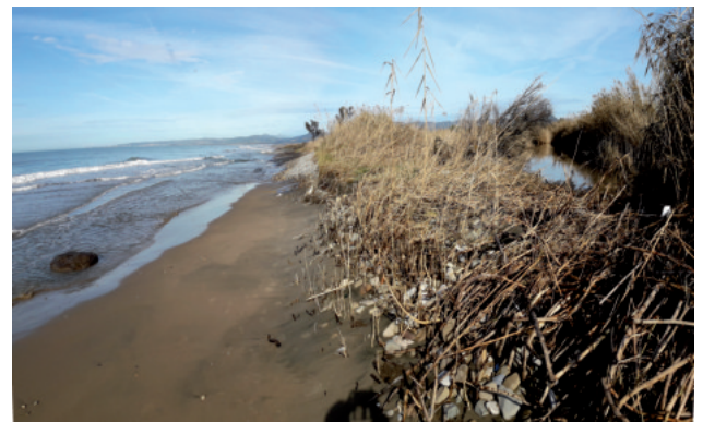
Fig. 7 - View of present damaged dune
