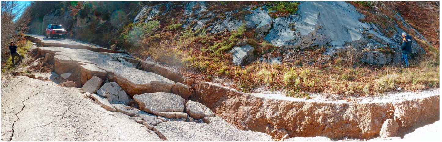
Figure 1. The impressive 30 October 2016 surface faulting along the antithetic San Lorenzo Fault. Here the fault crossed and destroyed a dirt road, with an offset of ~1 m. Note the rock-fault scarp that crops out just above the coseismic free-face (right side; car and persons for scale). Photo taken 3 hr after the earthquake.
