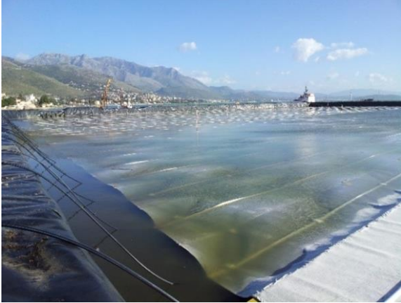
Figure 1. Horizontal drains and connections with the vacuum pumps circuit (de Lillis and Miliziano, 2016).
