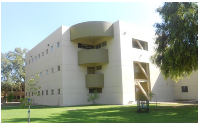
Figure 2: New three floor building of the IoE.
