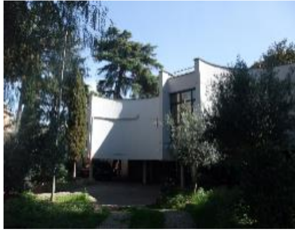
Figure 6. Church of Santi Martiri dell'Uganda, the entrance of the Rectory from the garden.
