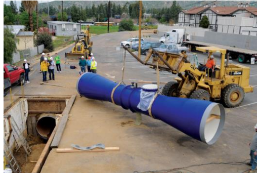
Fig. 8. Lucidpipe installation in Riverside, California.
