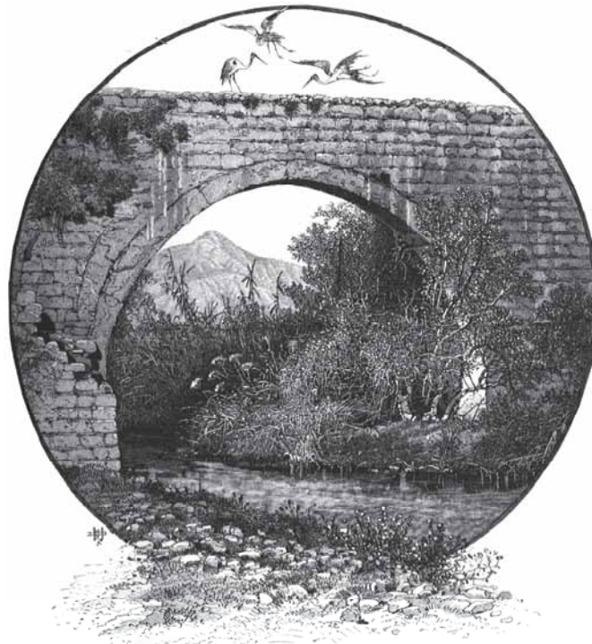
Fig. 2.4 - Aqueduct over the Wadi Oelt at the end of the 19 th century (after C.W. Wilson, Picturesque Palestine, Sinai and Egypt , p. 169).
