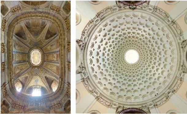
Figure 10- Zenith views of the ceiling of the churches of Santissimo Sacramento or Oratorio dell'Angelo Custode (on the left) and of San Bernardo alle Terme (on the right).
