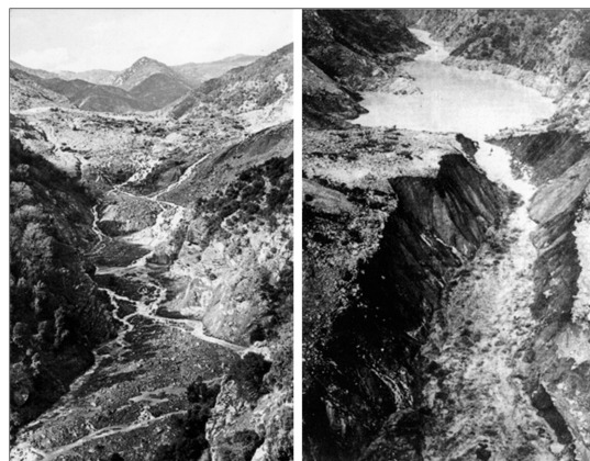
Figure 2. Photos taken immediately after the landslide events of January 1973. On the left the Bonamico river valley, on the right the diffuse erosion along the Costantino Lake outflow and on the landslide dam body. Photos taken from [49] (used with permission of the copyright holder).
