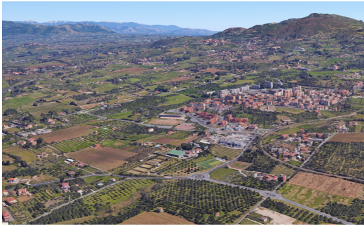
(a) Aerial View (Source: Google Earth)
