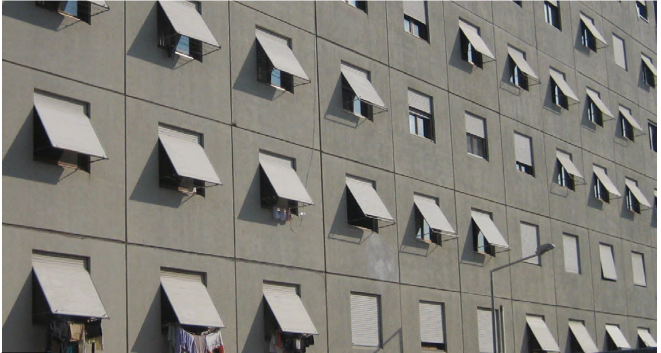
FIG. 26 A building of the district of Valmelaina (N 6), the repetitive sequence of parallel r.c. wall enhanced the semantic of loculus , clearly shown here also in the façade envelope cladding panels
