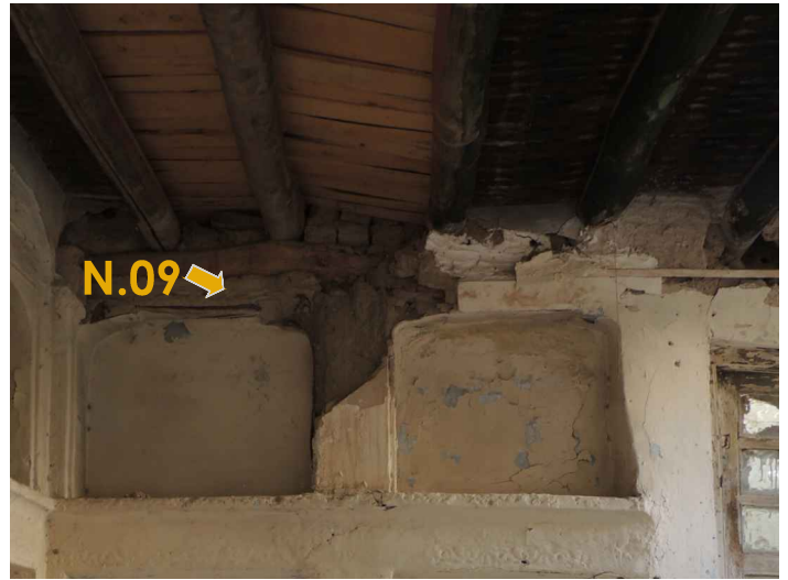
Nili's house, first floor, guest room, northeastern wall.
