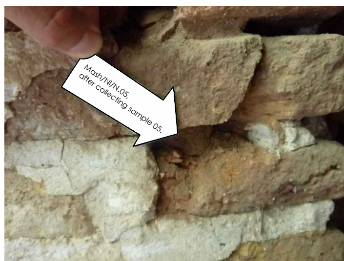
Nili's house, southwestern section, ground floor, after collecting sample Mash/NI/N.05.
