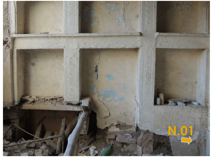
Nili's house, first floor, guest room, southwestern wall.
