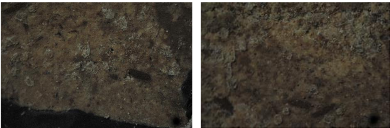
Figure 3.20 Burnt brick sample collected from Bidari House, NE building mass, ground floor, living room, western wall. 157
