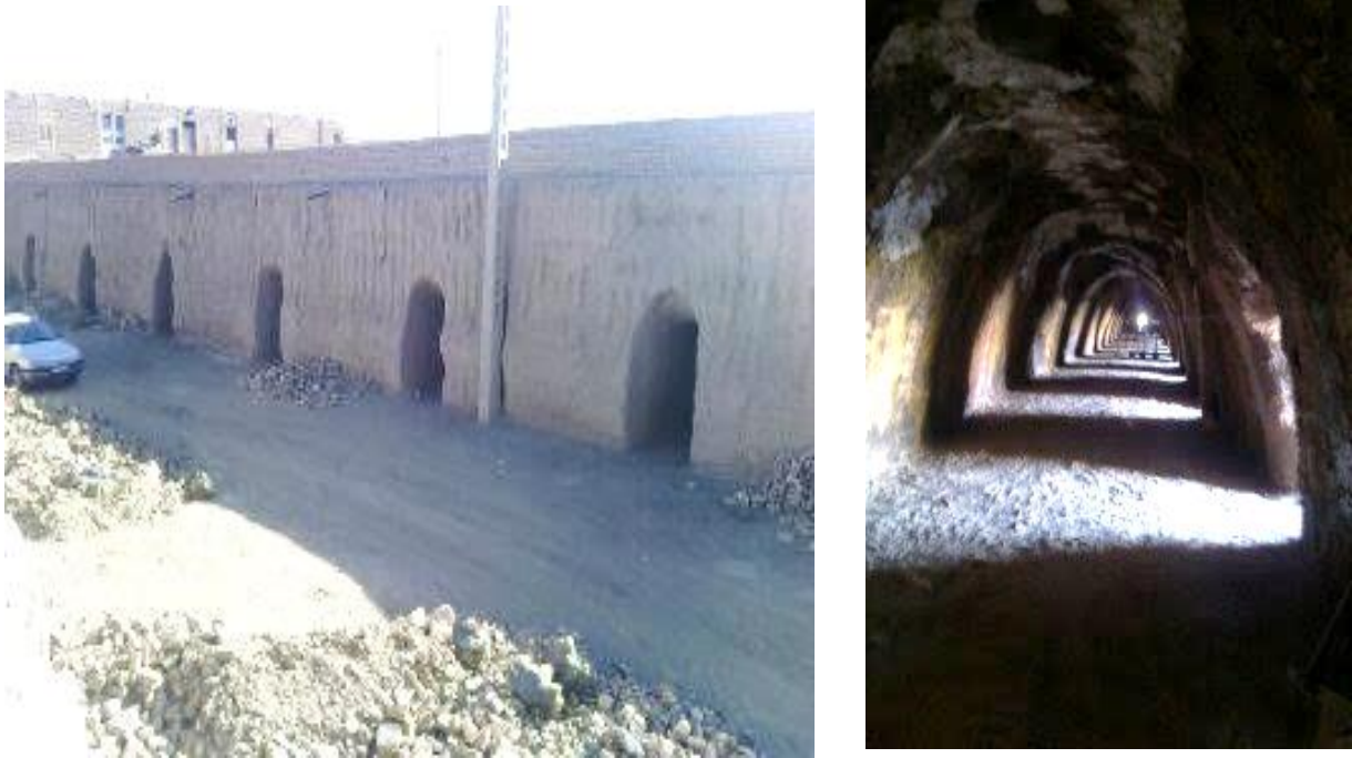
Figure 3.10 The Hoffman kiln near Gonabad (284 km to Mashhad) which serves as a traditional kiln to produce the bricks used for restoration of monuments
