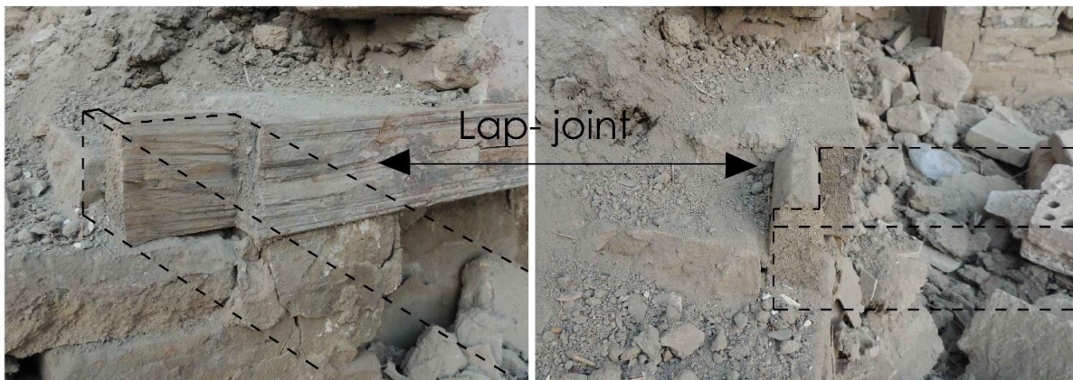
Figure 3.3 Connection of horizontal beams by lap-joints in the ground floor of Bidari House. (After the building demolition, 2017)
