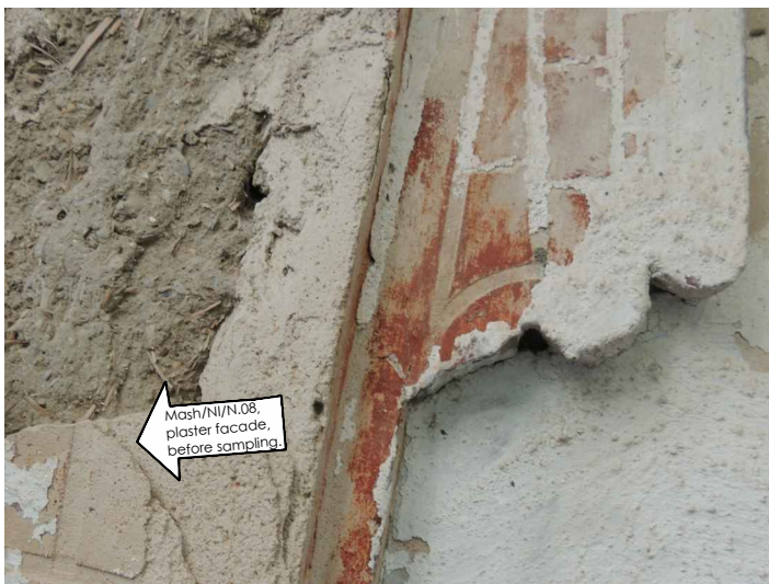
Nili's house, southwestern facade, MASH/NI/N.08. Sampling of plaster facade.
