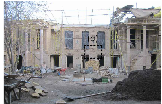
Fig. 4.13.1 The southeastern building mass in the last phase of the restoration.
