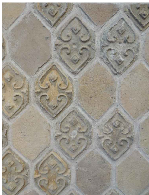
Fig. 4.13.3 Reconstructing the damaged part of the walls with recycled bricks that are the same in terms of shape and size, avoiding the use of bricks that have the geometric pattern to highlight the two types of material, reused and original.
