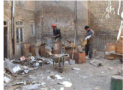
Fig. 4.1.2 Emptying the courtyard and rooms from garbage and waste.
