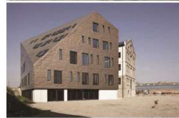
Pollard Thomas Edwards Architects, The Granary Barking , Londra (2011)
