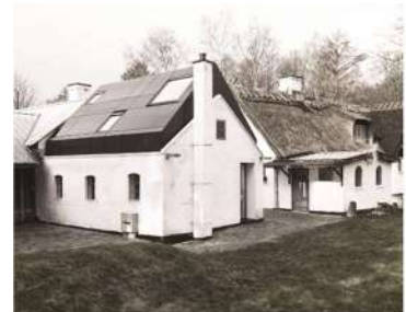
Svendborg architects, Studio POSEhuset , Farum, Danimarca (2010)
