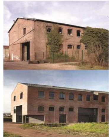
H2O ARCHITECTES, Business incubator Training centre «La Cartonnerie», Pont-Audemer, Francia (2014) foto: Attard, Chalmeau
