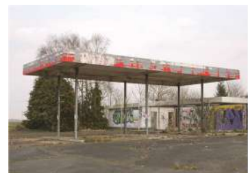
Foto da “ Twentysix Recycled Gasoline Stations ”, Eric Tabuchi (2010)
