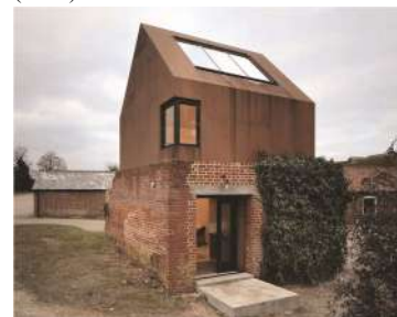
Haworth Tompkins Architects, Dovecote Studio, Suffolk (2009)
