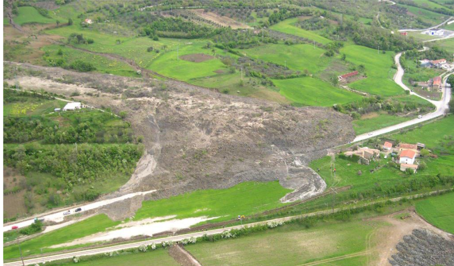
Figure 18 - Landslide toe covering the National Road SS90 after 2006 movement (source: Guerriero, Revellino, Grelle, et al. , 2013)
