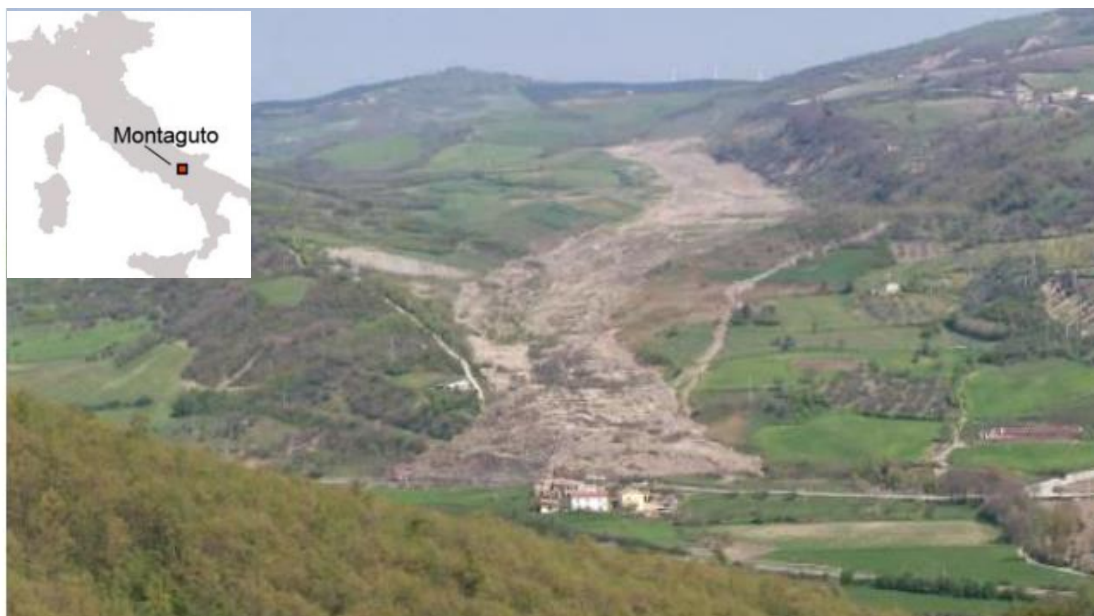
Figure 17 - Landslide body and run out after the reactivation in 2006 (source: Cascini et al. , 2012)
