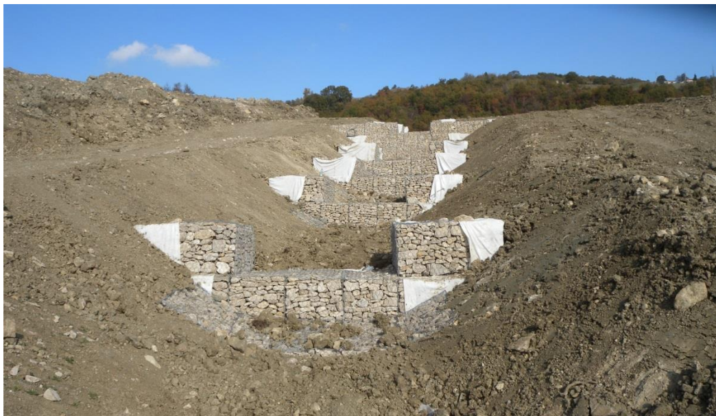
Figure 28 - Trench channel works
