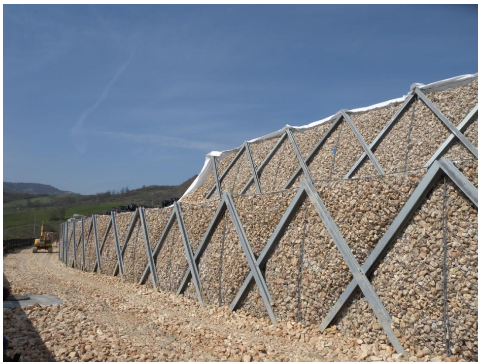
Figure 29 - Retaining gabions on the toe
