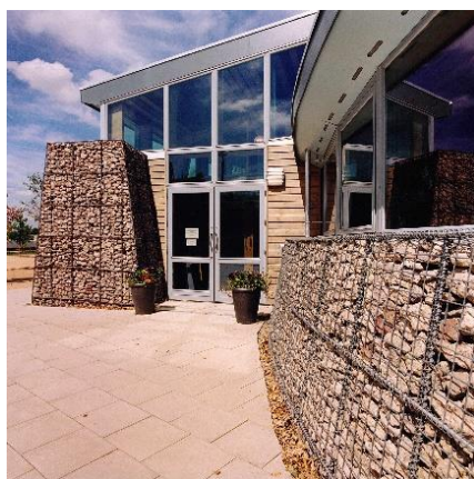
Fig. 108 Il Conference Building dell'Earth Centre e la Prayer room di Kwait City [Dernie, 2003, p. 53; http://www.enviromeshgabions.co.uk ]
