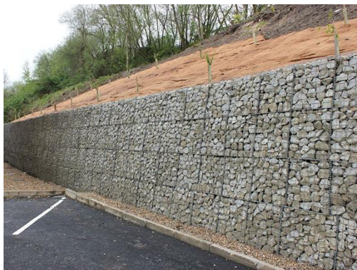
Fig. 64 Muro di contenimento a gabbioni (Royal Tunbridge Wells, Kent) [ http://www.hy-ten.co.uk ]
