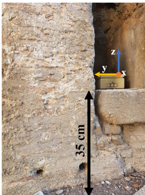
Figure 15 Placing of the measurement system at the third niche of Minerva Medica Temple at 35 cm.
