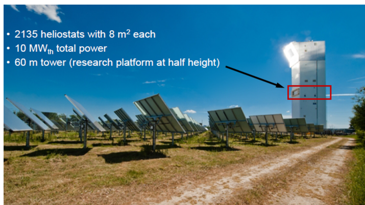
Figure 6.1: Solar tower and heliostates field in Juelich. Reference of picture: Thomey et al. [2016]
