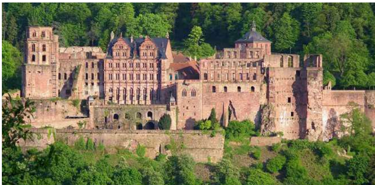
1. Vista del Castillo de Heidelberg** 1. View of Heidelberg Castle**
