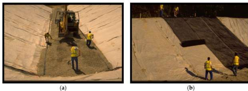
Figure 4. (a) Bottom and; (b) lateral watertight during the placement.
