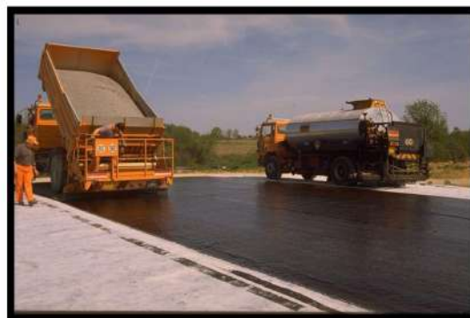
Figure 5. Placement of the 3-layer asphalt wearing.
