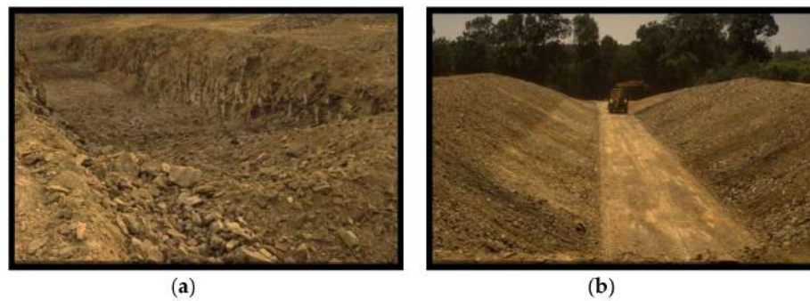
Figure 3. (a) Excavation of the mica schist ground support; (b) shape of the test site between embankments.
