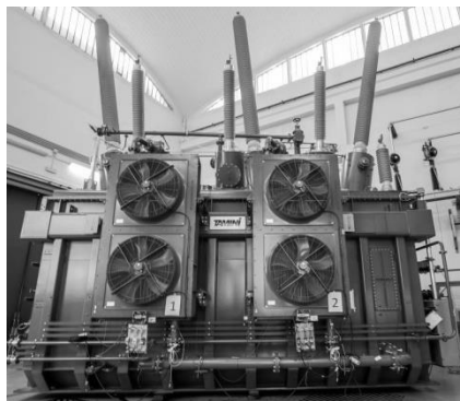
Figure 1: Tamini “green” transformer (ATR 15T037)
