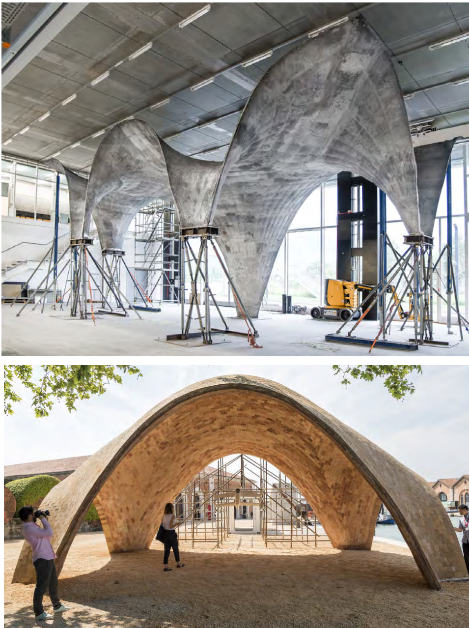
Figure 5. Block Research Group. Above: Construction prototype for ultra-thin concrete roof; Down: vaulted form made up from two layers of a new type of compressed earth blocks, Durabric, developed by the LafargeHolcim Foundation for sustainable construction.
