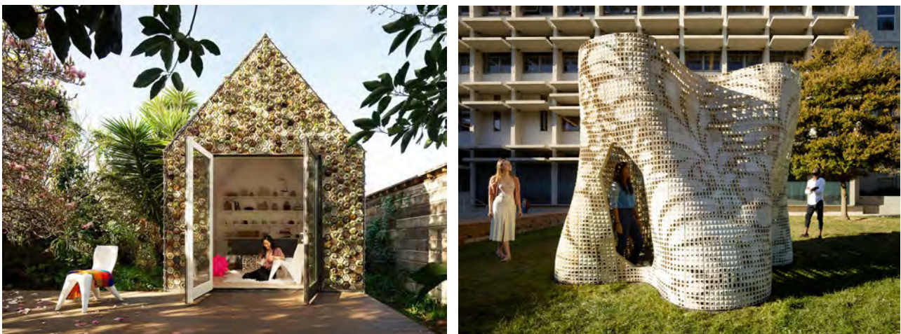
Figure 7. Ronald Rael and Virginia San Fratello, Emerging Objects: “Cabin of Curiosities” (4.500 ceramic tiles) Oakland, 2018; “Bloom Pavillion”, 3D print cement (This structural system was inspired by the Iglesia Cristo Obrero of Uruguayan architect and engineer Eladio Dieste and Jefferson’s serpentine brick walls at the University of Virginia, while the precise form was inspired by Richard Serra’s Torqued Ellipse .)
