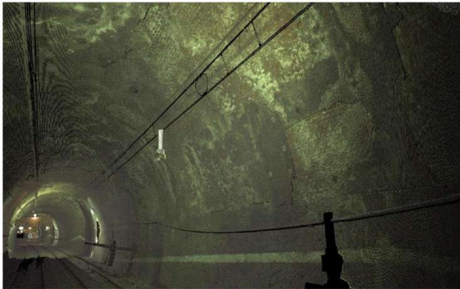
Figure 1. Image of a railway tunnel obtained through laser scanning technique.
