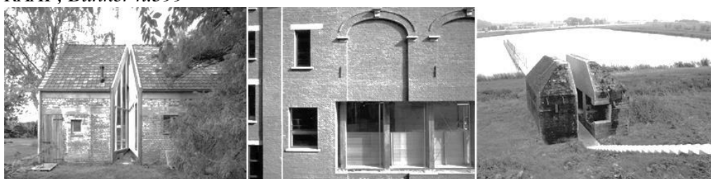
Figure 8. Jump Cut: (a) Advvt, Melle-matta House / (b) 51N45, Lamot Center / (c) RAAF, Bunker n.599
