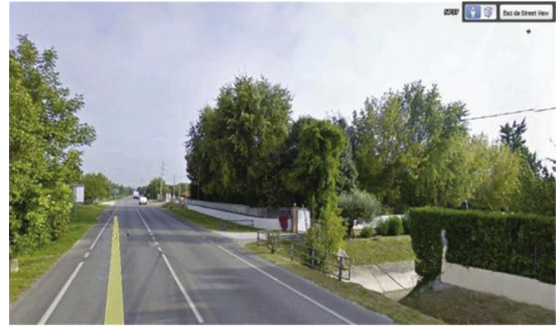
Fig. 4 – Presence of defects SB2 (present but inadequate safety barriers), SB3 (singular point of safety barriers), and CO4 (ditch).
